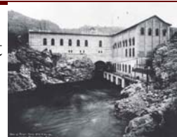
Rear of Lower Bonnington power house - W.K.P. & L. Co
